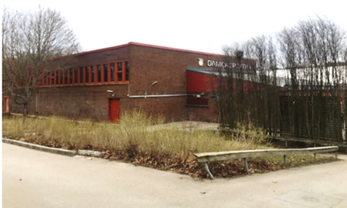
Futur Pension Sporthalls norra fasad (f.d. Danica sporthall).
